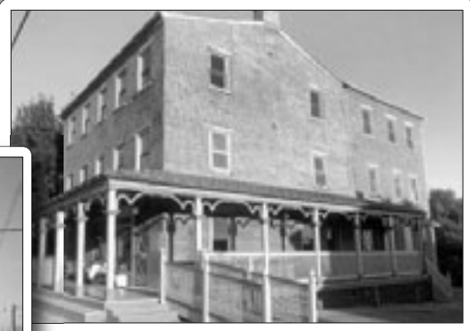
After: Iron Horse Inn/Hotel Strasburg, built Circa 1875. Wrap-around porch rebuilt 2005.
